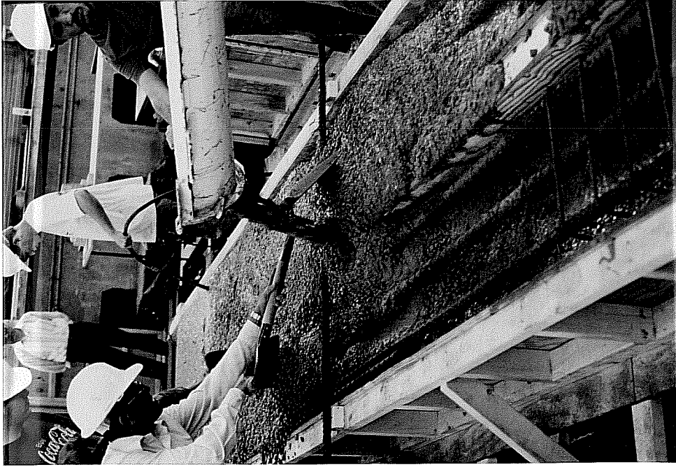
Figure 2.9: Casting - Series 1 (Ready-Mix Truck)
