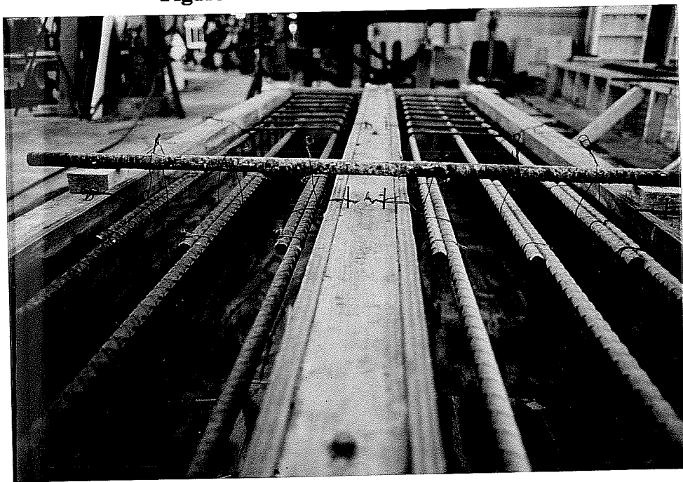
Figure 2.8: Splice Support Rod
